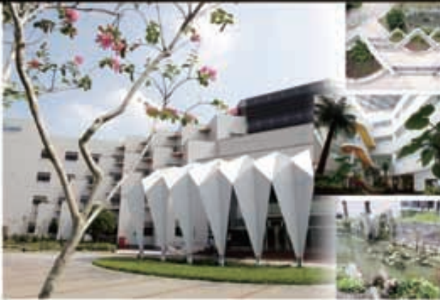
Green Building, Tainan Plant, Taiwan
